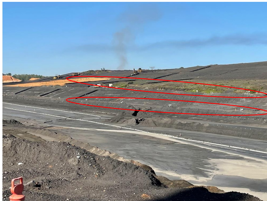
Figure 5. Deep wells on benches on a CCR slope. The upper and lower rows of wells are highlighted by the red ovals.
