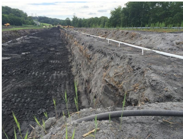
Figure 1. Wellpoints dewatering an excavation cut in CCR.
