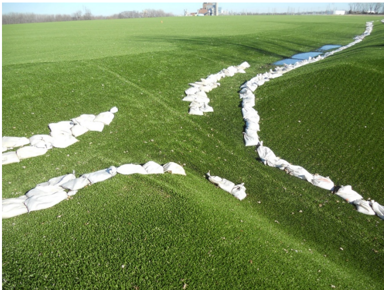
Figure 1: Perimeter ditch channel with ClosureTurf™.
