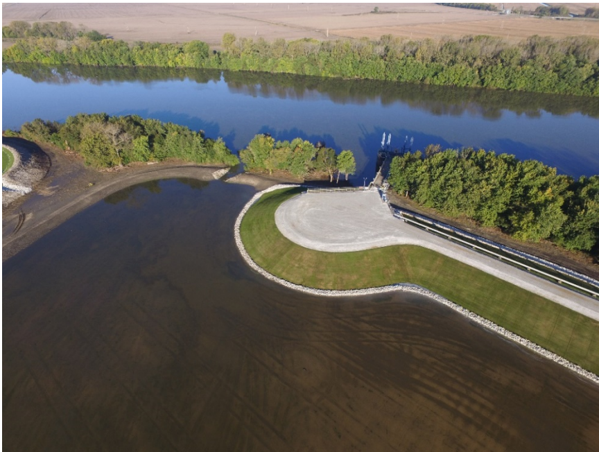
Figure 6: Completed dock facility access road
