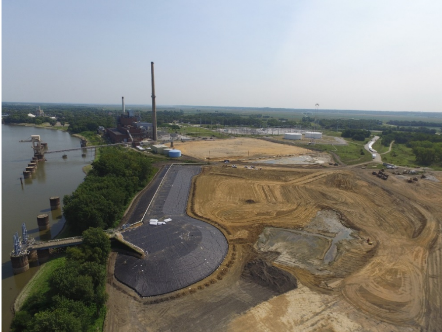
Figure 5: Dock facility access road (built upon CCR containment berm) during construction.
