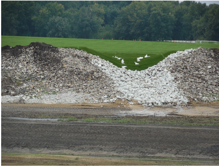
Figure 2: Energy dissipator at end of downslope channel.
