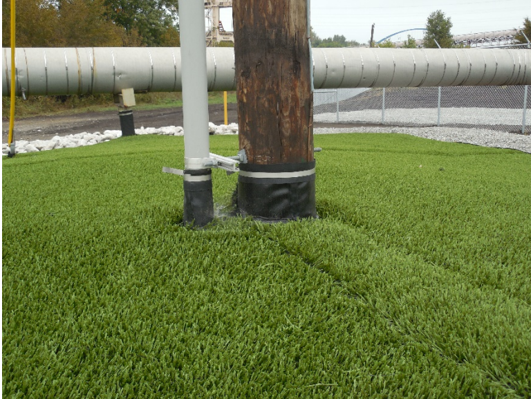
Figure 3: Geomembrane batten around utility pole.
