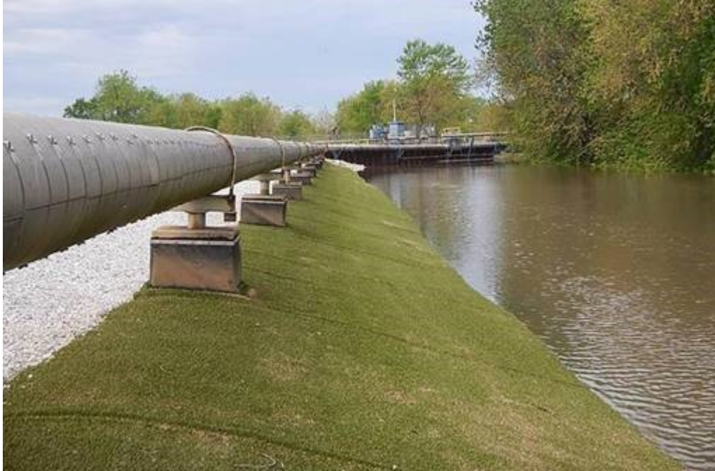
Figure 7: Flood waters on completed cap.
