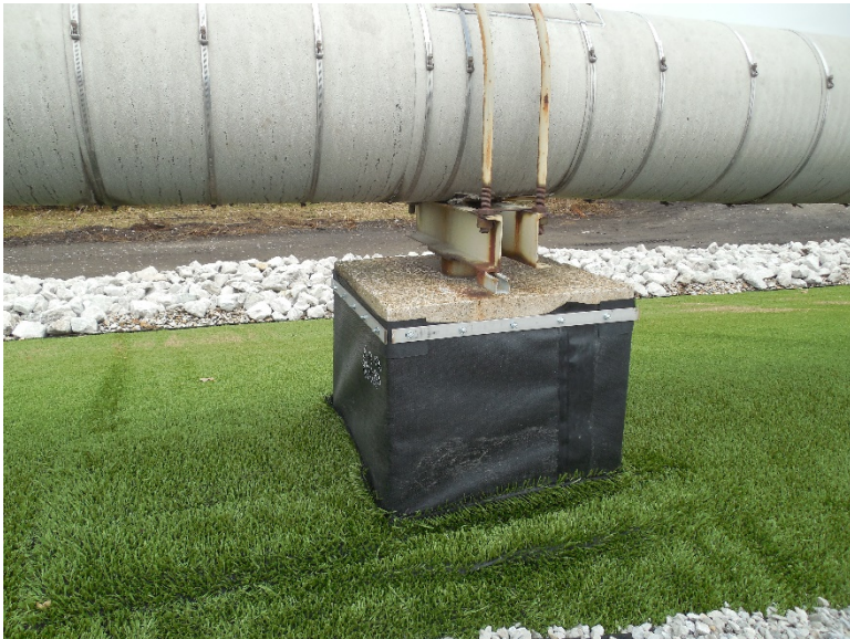
Figure 4: Geomembrane batten around pipeline foundation.
