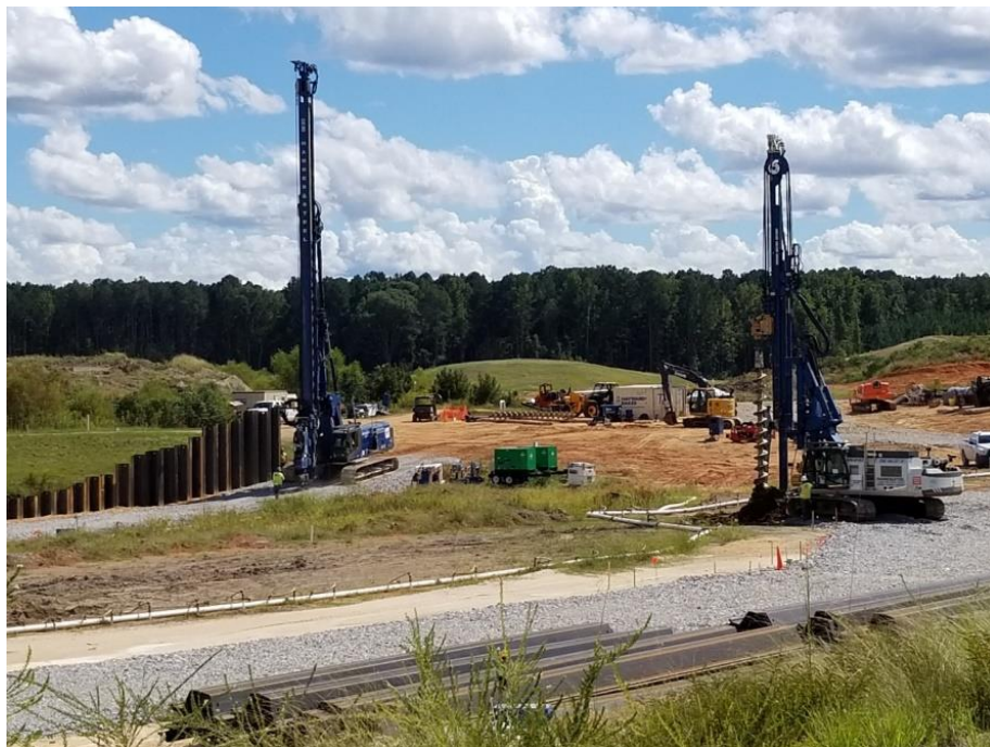
Figure 3. Equipment utilized for the installation of the earth retention.
