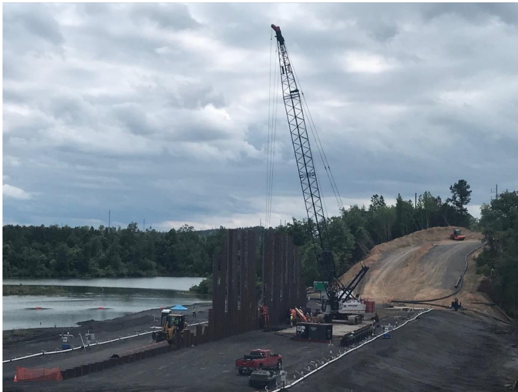
Figure 4. Using a crane on ash to drive sheets.
