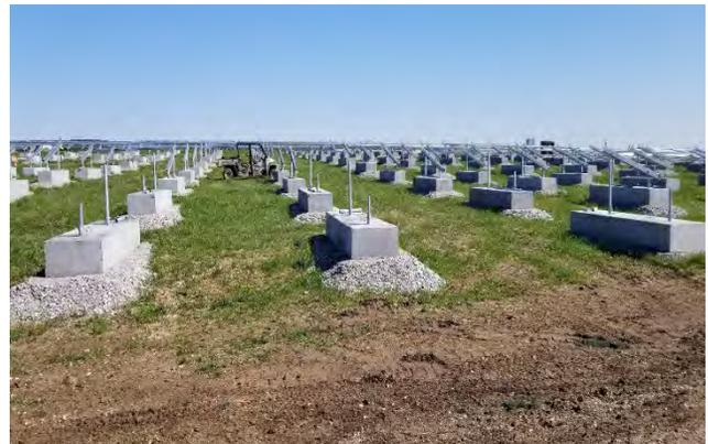
Ballast systems and equipment pads can either be pre-cast or constructed on-site. Both require some movement of materials by equipment that will wear on the turf cover. The same is true of setting inverters, but much of the rest of construction is conducted manually. Placing these structures on
